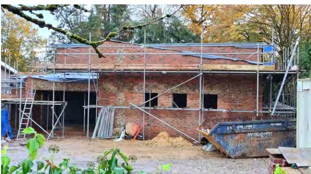
Progress of the Cornerstone project (rear view above, front view below)
